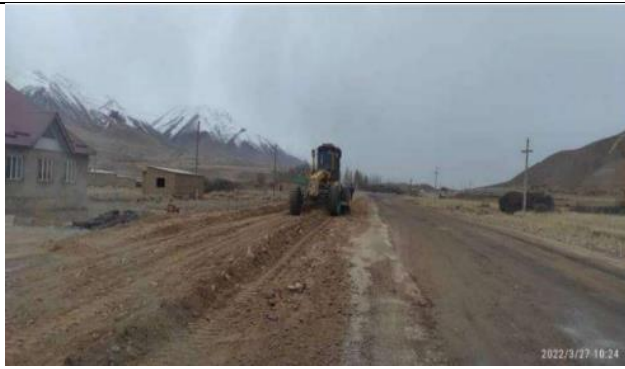
Фото 21. Construction of embankment at Km 89+340.
